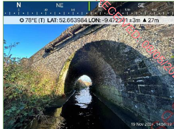
Plate 3.7d Single barrel stone bridge at WC#3.
