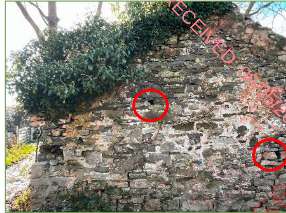
Plate 3.9b Gable end of the stone structure, highlighting two crevices suitable to support individual roosting bats occasionally (S_09).
