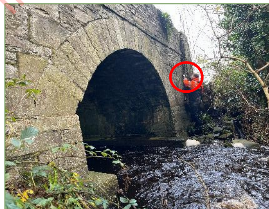
Plate 3.6b The south facing spandrel wall within which a crevice was discovered and deemed to be of 'Low' suitability.
