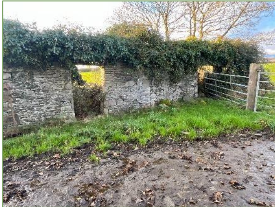
Plate 3.9a Remnants of an old stone farm building 'S_09'.
