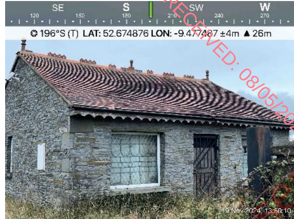
Plate 3.13a Unoccupied single storey stonework building (S_11).
