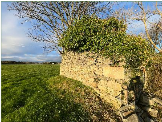
Plate 3.9c Gable end of the stone structure, with suitable crevices and moderate Ivy cover (S_09).
