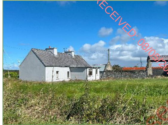
Plate 3.3 Residence (S_03), stone structure (S_04) and other farm buildings (S_05).
